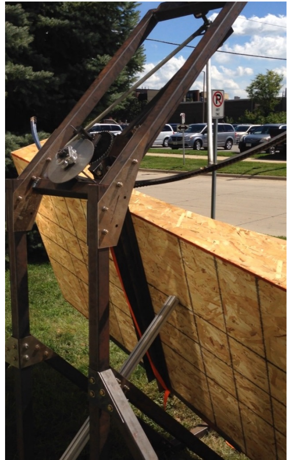
Figure 4.6: Completed Tracking Stand
